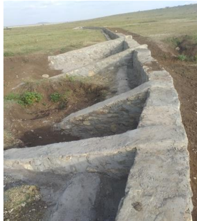
Illustration 1: a WSW spreads water and its sediment and reduces the velocity of water flow by enhancing the length of the water way
