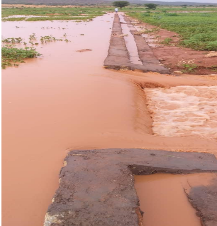
Illustration 1: a WSW spreads water and its sediment and reduces the velocity of water flow by enhancing the length of the water way
